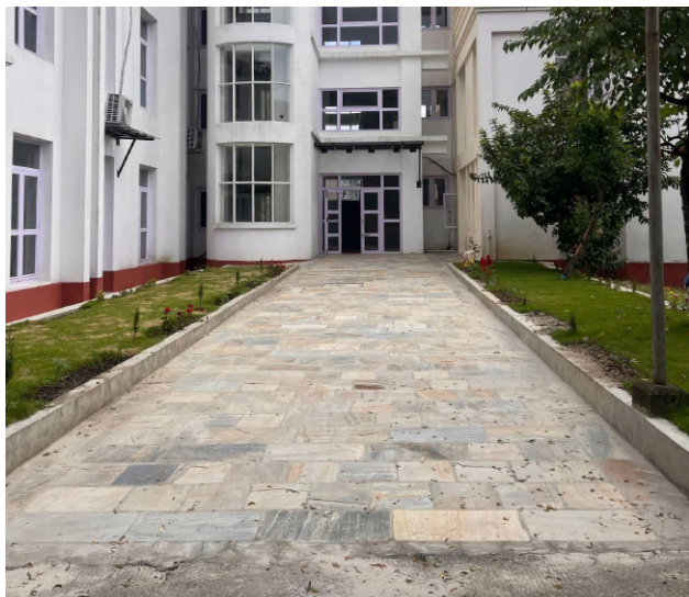
Newly Constructed Walk-way at Sampada Sadan
