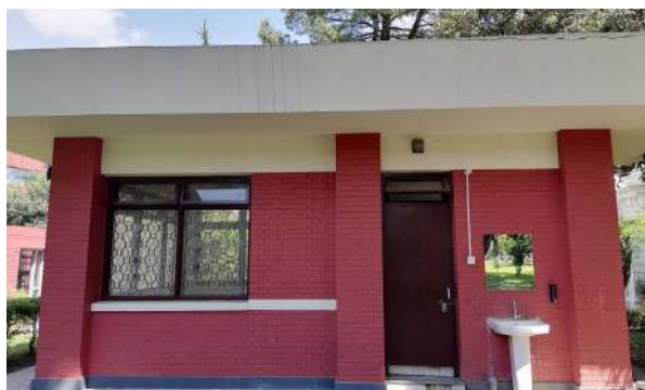
Renovated Guard House
